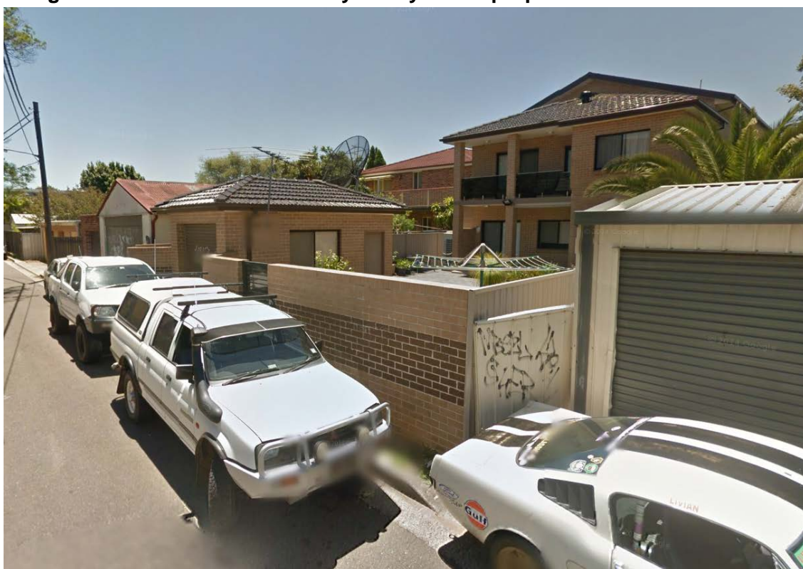
Figure 3 – View of rear boundary of Lily Street properties from Roberts Lane
